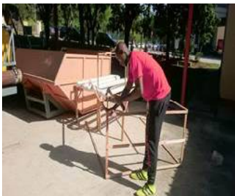
e) Assembling ceiling wood for net protection/awning.
