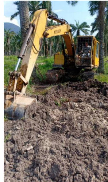
Figure 1 Excavator bucket tilting the soil
