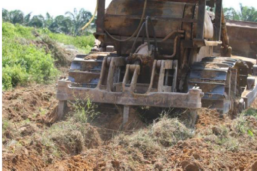
Figure 4 Fabricated ripper on D6 bulldozer ripping the soil
